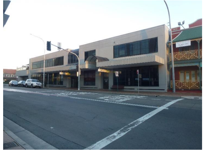
Figure 16: Two storey commercial building at the intersection of Scott and Terminus Street
