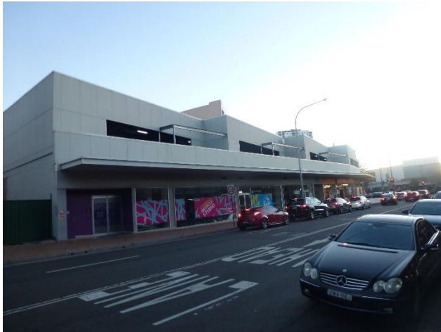
Figure 4: Commercial building occupying the site as viewed from Scott Street (north east)
